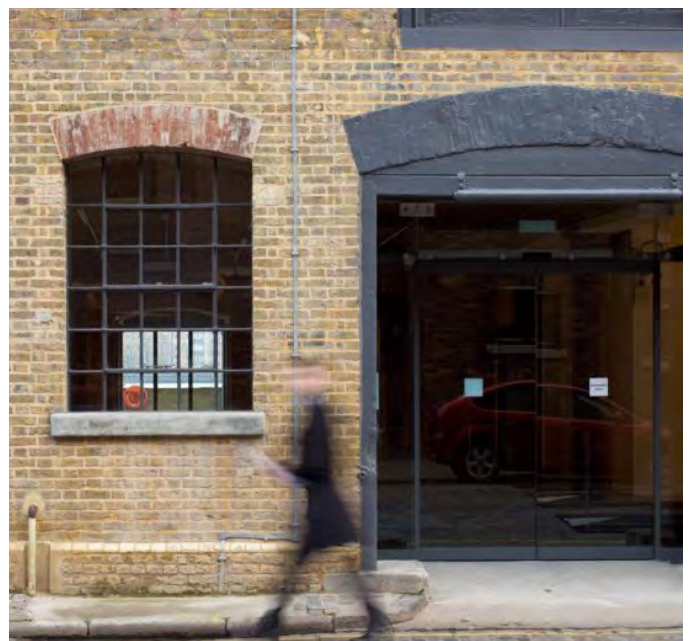
Fig.545 Metropolitan Wharf, London
