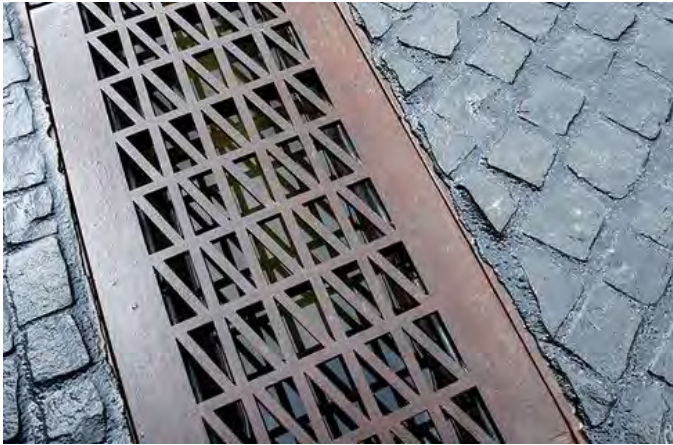
Fig.367 Iron channel drain
