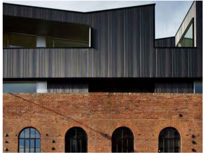
Fig.425 Metal sheeting, Shoreham Street, Sheffield
