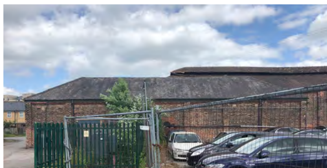
Fig.254 Albion Iron Foundry shop - parallel brick shed - west facade
