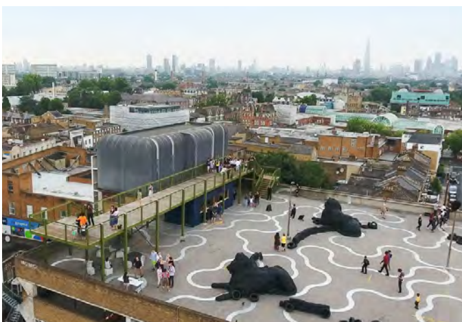
Fig.568 Bussey building roof top cafe sculpture park, Peckham
