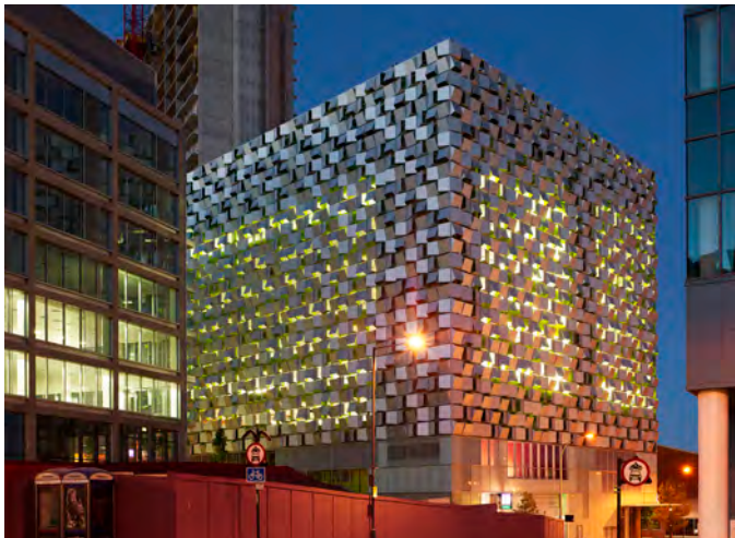
Fig.429 Carpark structure, Charles Street, Sheffield
