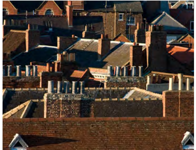
Fig.294 Existing York roofscape variety
