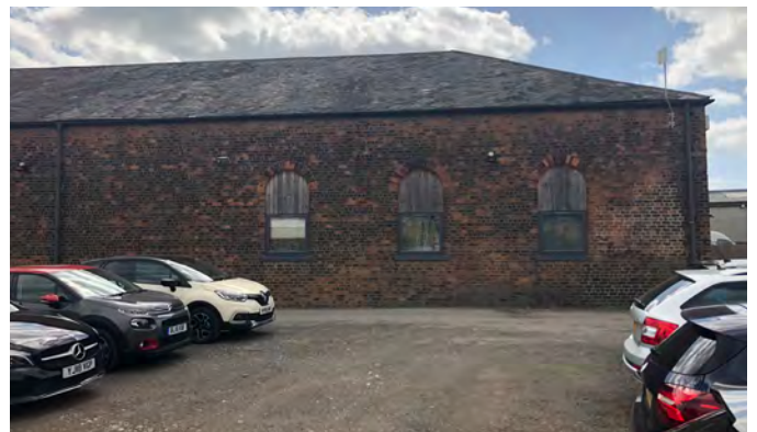
Fig.257 'Engine Shed' north facade east facade
