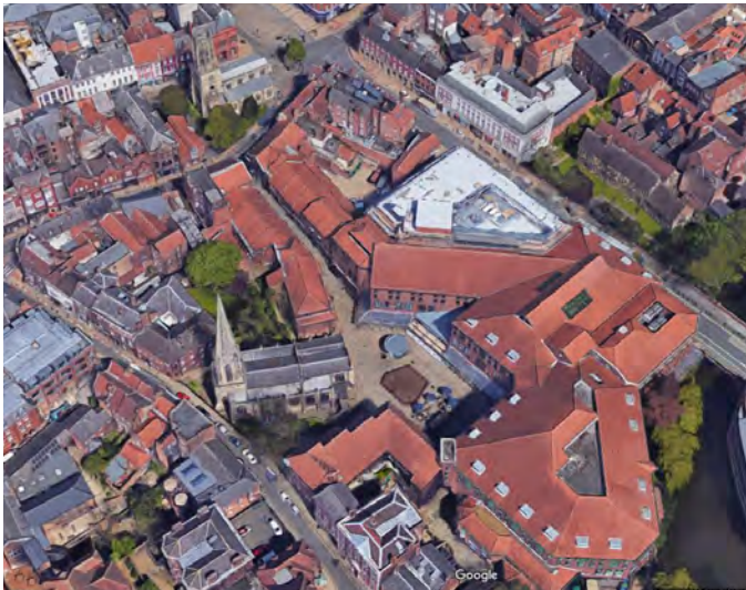
Fig.289 Large scale clay tiled roof to Coppergate shopping Centre ❌
