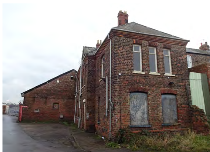
Fig.259 East frontage of Smith's Shop Office
