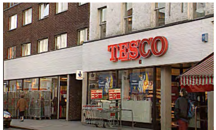
Fig.356 Shopfront fascia dominates building
