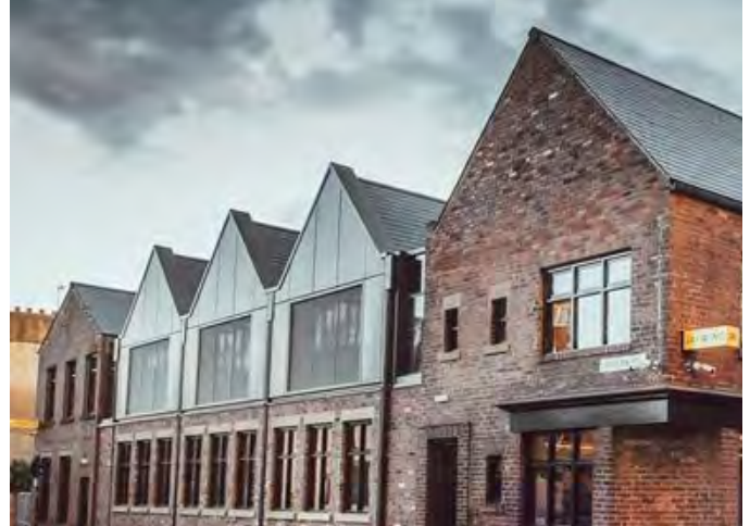
Fig.235 Example of contemporary extension to an industrial heritage asset (Albert Works, Sheffield)
