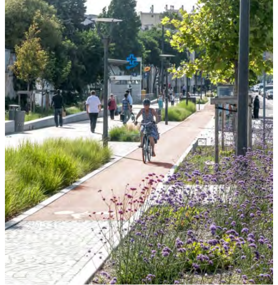
Fig.125 Dedicated cycleway, France
