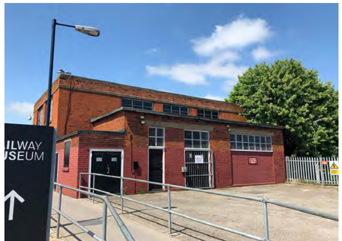
Fig.269 Generator building seen from the east
