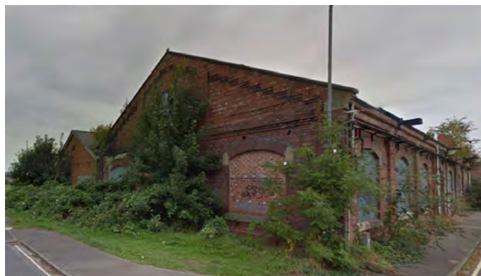
Fig.271 Carriage works mess room
