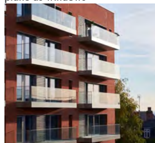
Glass balustrade to projecting balconies ✗
