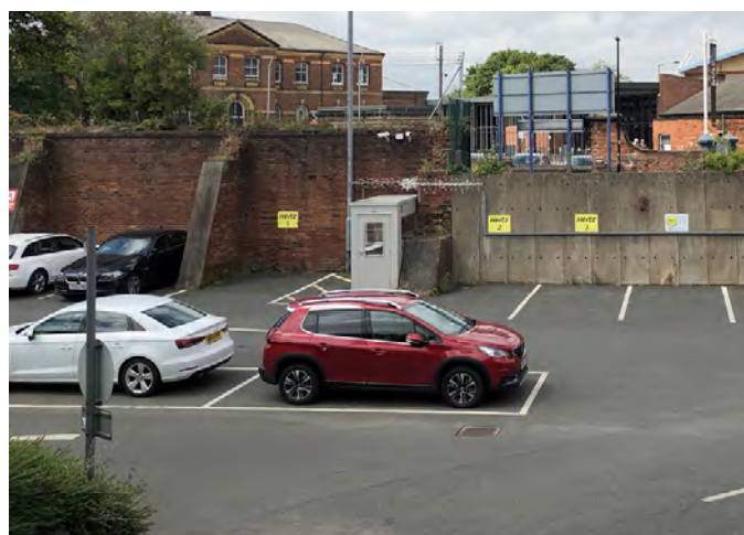
Fig.265 East face of the Coal Drops with the National Railway Museum beyond
