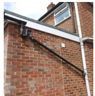
Fig.314 Ill-considered downpipes
