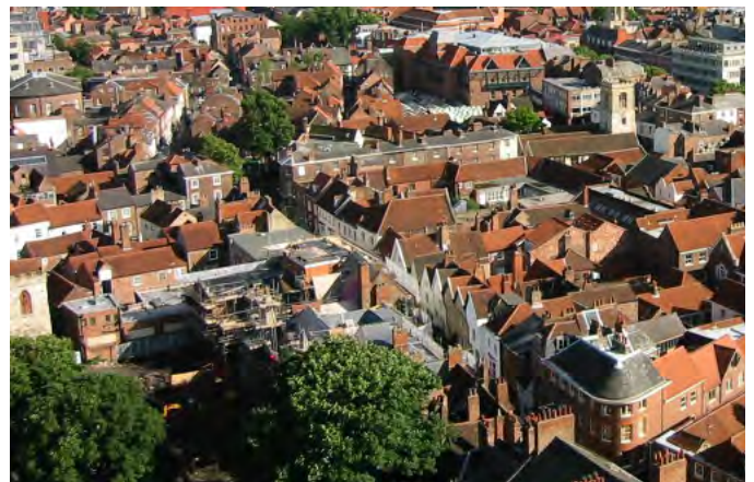
Fig.295 Existing York roofscape variety
