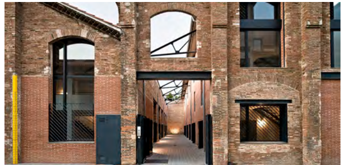
Fig.236 Example of contemporary interventions in brickwork (Seta Bonet architects)
