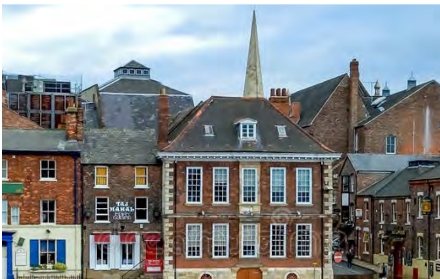
Fig.333 The colours of masonry walling in York Central shall follow a similar palette to the existing in the historic city
