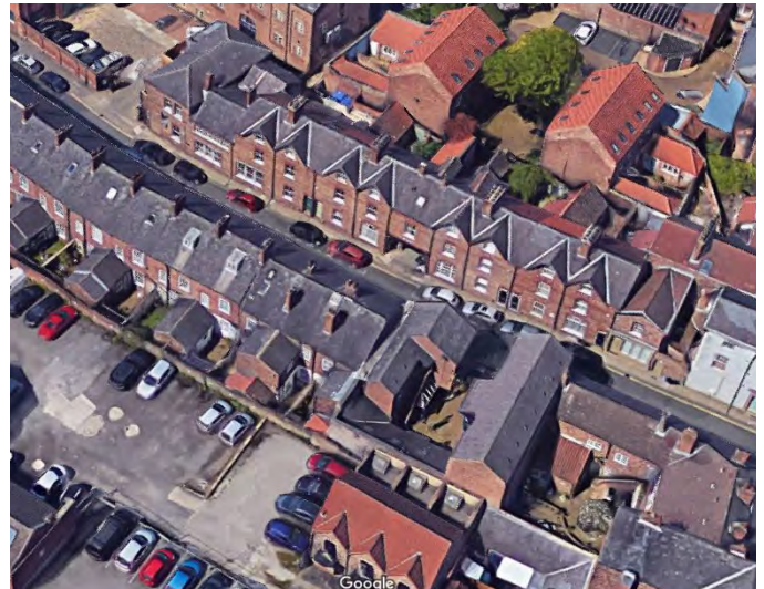
Fig.292 Small scale roofs to houses on George Street ✔️
