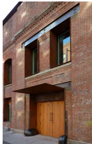
Fig.237 New windows and entrance at the Eberhard Faber Pencil Factory, Brooklyn
