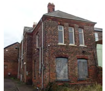
Fig.483 Smith's shop office
