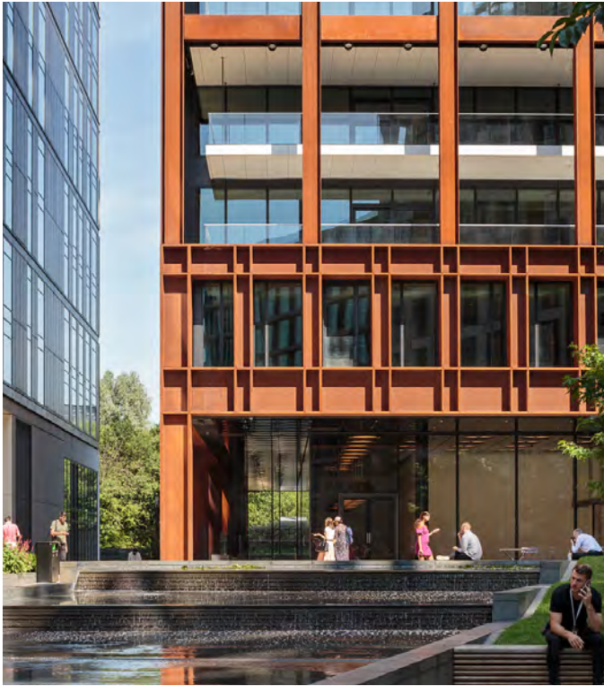
Fig.546 St Pancras Square, Kings Cross, London
