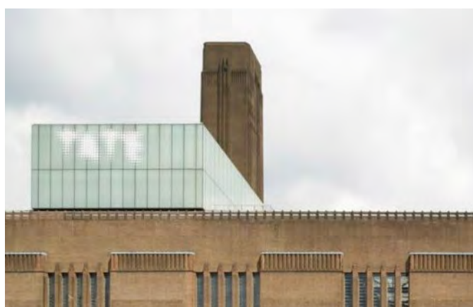
Fig.262 Example of a roof extension in material contrasting with the brick base
