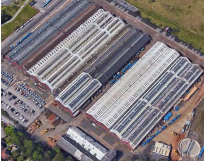
Fig.288 Very large scale, repetitive industrial roofs ❌
