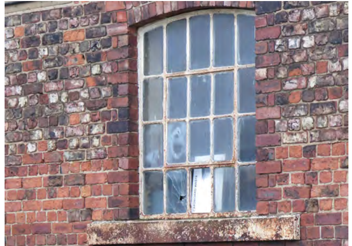
Fig.246 Existing iron window could be retained and repaired
