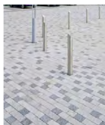
Precast concrete - small units
