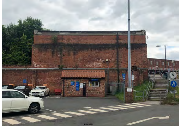
Fig.268 Generator building seen from the west
