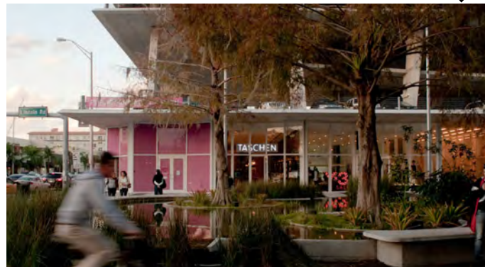
Fig.436 Car park with open active facade
