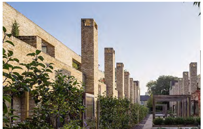
Fig.296 An example of good contemporary chimney design in Accordia, Cambridge
