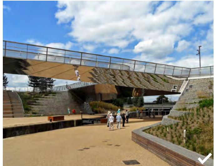
Fig.91 Olympic Park, Stratford, London
