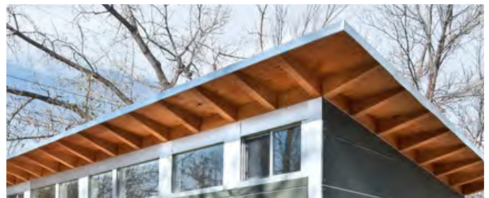
Fig.310 Example of a contemporary eaves detail
