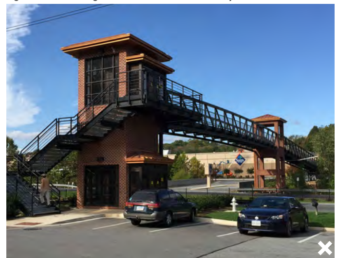
Fig.93 Example of inappropriate pedestrian crossing
