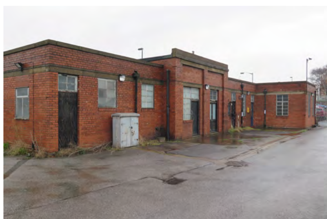
Fig.261 South elevation of 1930s Leeman Road building
