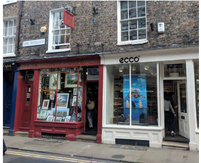
Fig.354 Examples of York city centre shopfronts
