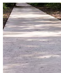
In-situ concrete with exposed aggregate
