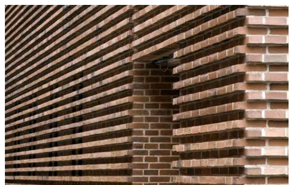
Example of a deeply articulated brickwork giving texture and depth to a facade surface
